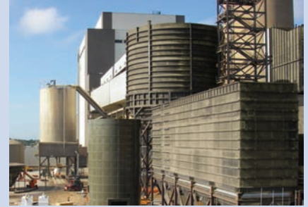
Bolted RTP, Field-weld & Hybrid Tank Construction
